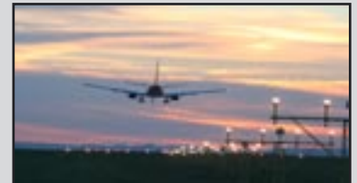
Measuring airfield guidance lights
