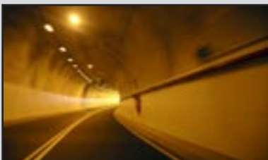
Lighting of tunnels
