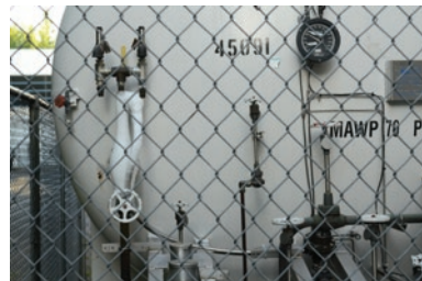
Difficult inspection sites
