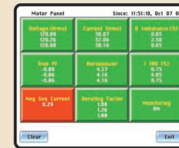
Unique annunciator screen collects and analyzes a range of motor health parameters to provide advanced warning of factors that could impact motor efficiency and performance.
